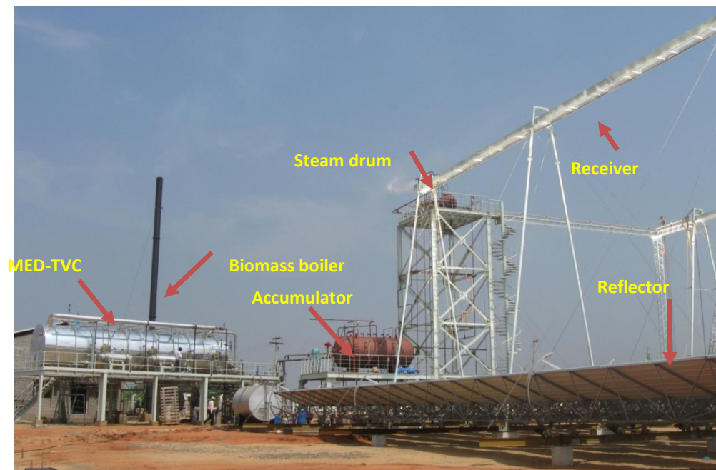
Fig.3 Overall view of the Solar field, MED and biomass boiler in Solar Desalination Plant
